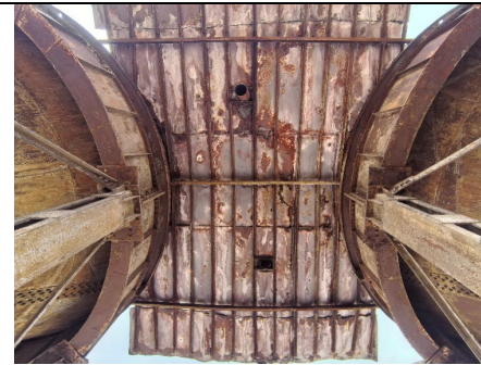
储料双罐中间钢雨棚
